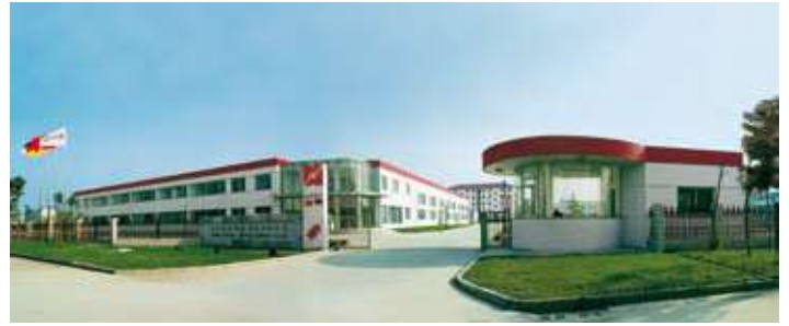
Nanjing works, productions facility to serve the Chinese market
