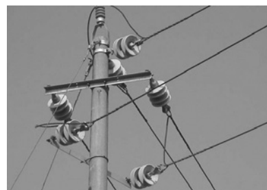
Dead-end for AAC conductor
