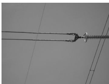
Dead-end for ACSR conductor
